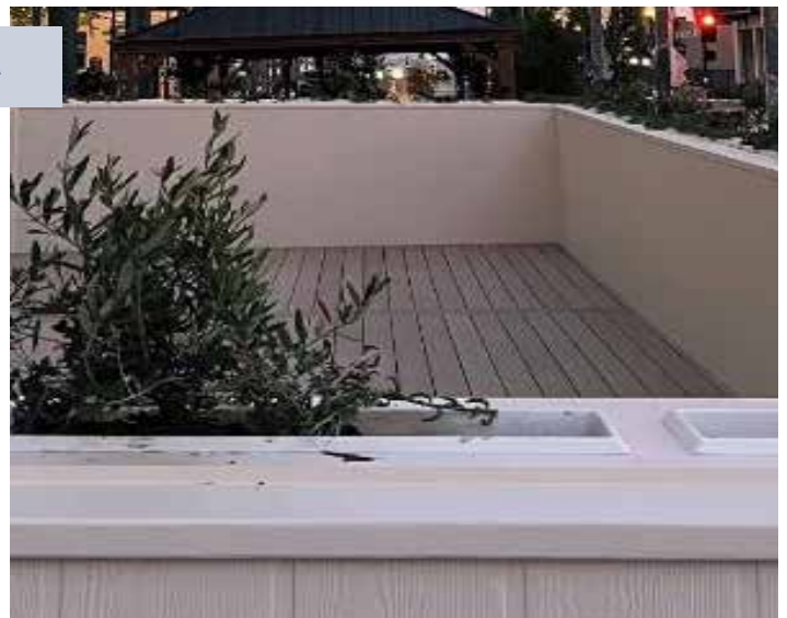
Example of a fortified parklet in construction in the MSM area with a heavy water-filled barrier and planter covered by a solid wood panel
